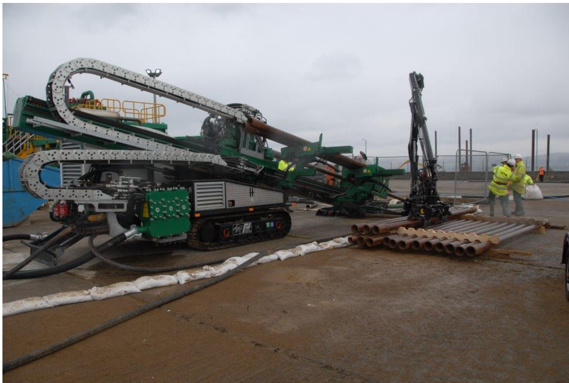
Plate 1: Typical Horizontal Directional Drilling Rig
