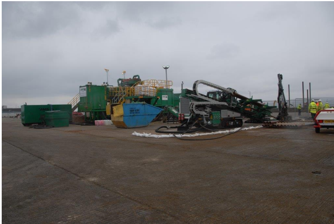
Plate 14.2.2 Typical Mud Handling Plant (located to rear of the drilling plant)
