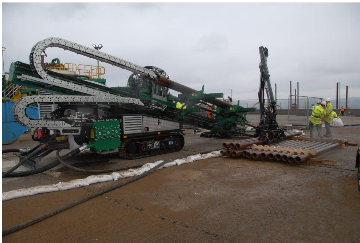
Plate 14.2.1 Typical Horizontal Directional Drilling Rig
