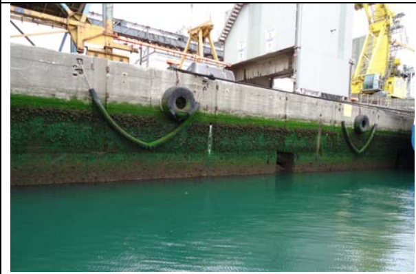
View looking N along Alexandra Quay, showing the mass concrete façade that defines its construction from the 1920s
