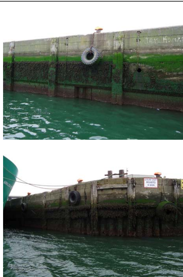
Views looking E (top) and NE (bottom) of Ocean Pier, showing its mass concrete construction of 20th-century date.
